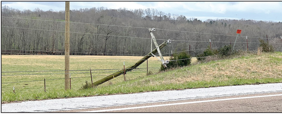
At least two electrical poles were blown down last Tuesday. TVEC employees worked hard to restore power to customers as quickly as possible.
